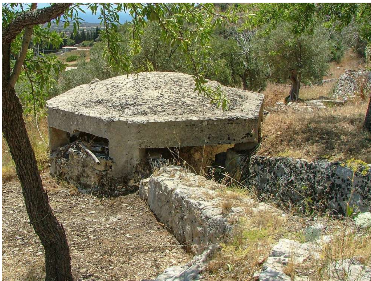
A hexagonal concrete casamatta with at least two longish machine-gun portholes and an entrance protected by a shallow wall [source: Lorenzo Bovi].
