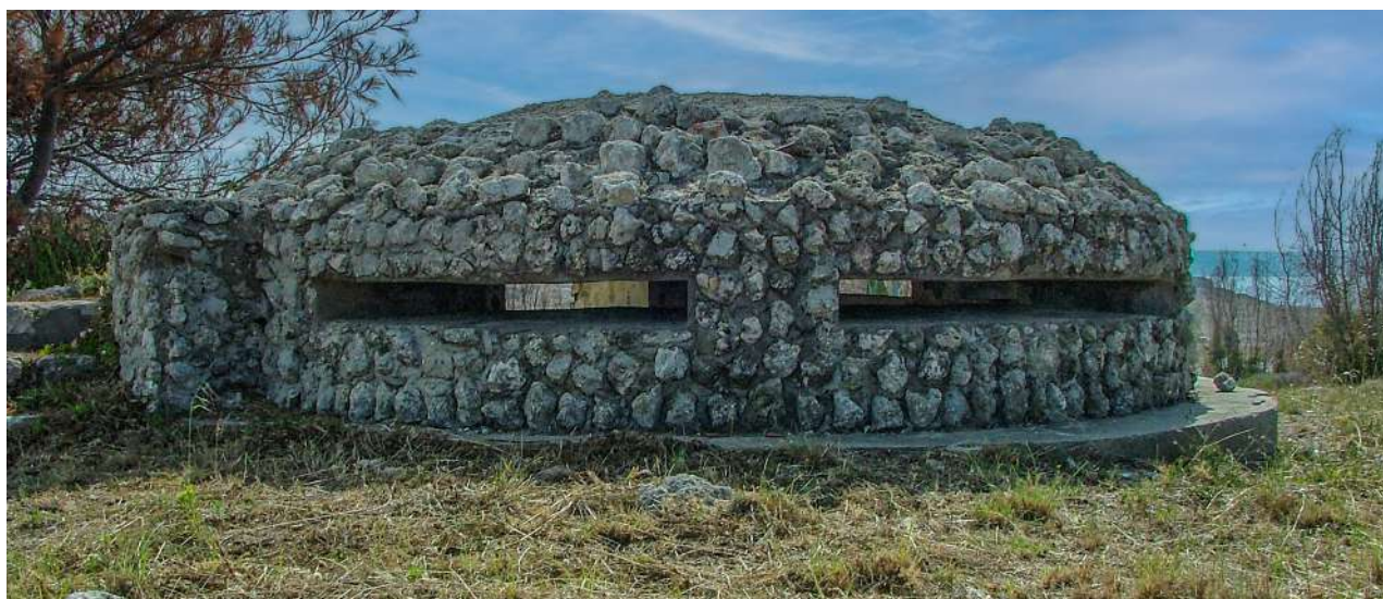
One of the casamatte at forming part of the Cozzo Telegrafo complex at Brucoli Campolato with thin longish portholes for observation and machine-gun/s. It is clad with rubble stones. This defensive complex defended the stronghold of Augusta and Syracuse [source: Lorenzo Bovi].
