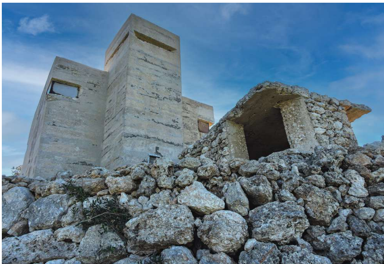
A squarish pillbox with a longish turret, four machine-gun portholes and a frontal searchlight emplacement at the foot of the same structure, at Il-Qortin tal-Iskrovitt.
