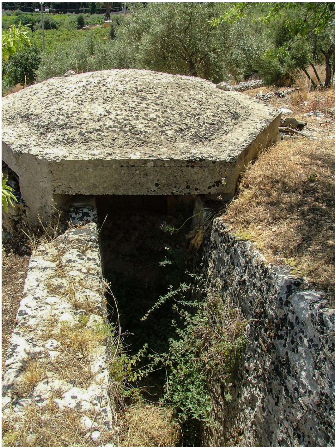
A close-up of the entrance to the same casamatta . Note that the wall is not shallow, but dug in earth, protected by a wall, as consigliament [source: Lorenzo Bovi].
