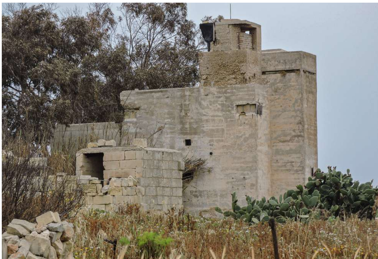
A squarish pillbox with a longish turret, four machine-gun portholes and a small searchlight emplacement at Benghisa, Birżebbuġa.
