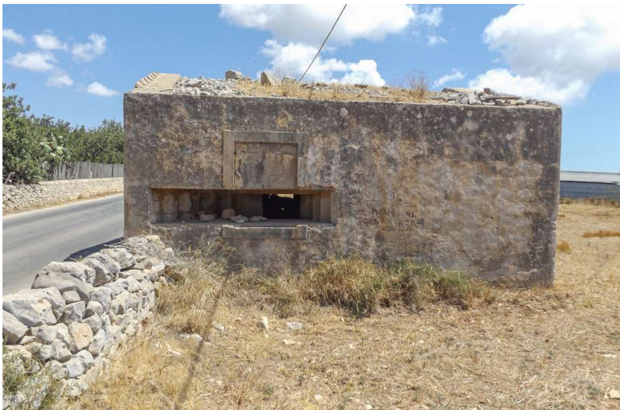
A rectangular casamatta with a longish porthole for a light anti-tank gun, at Punta Secca, Scicli [source: Lorenzo Bovi].
