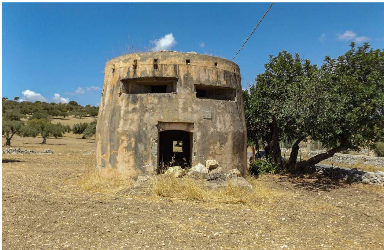
The rear of a casamatta , with an entrance and two machine-gun portholes at Punta Secca, Scicli [source: Lorenzo Bovi].
