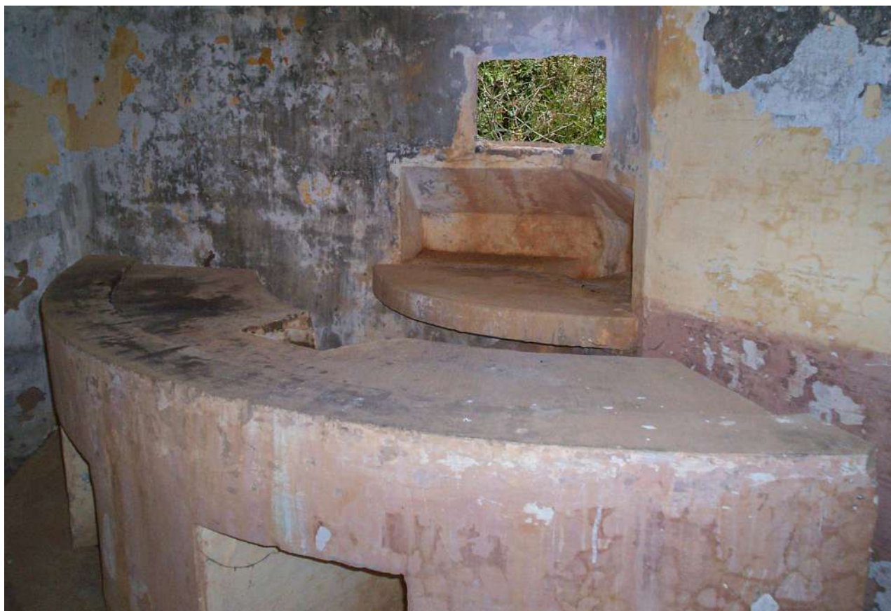
Inside the pre-war depth-post, with one of the concrete benches and a machine-gun port-hole.
