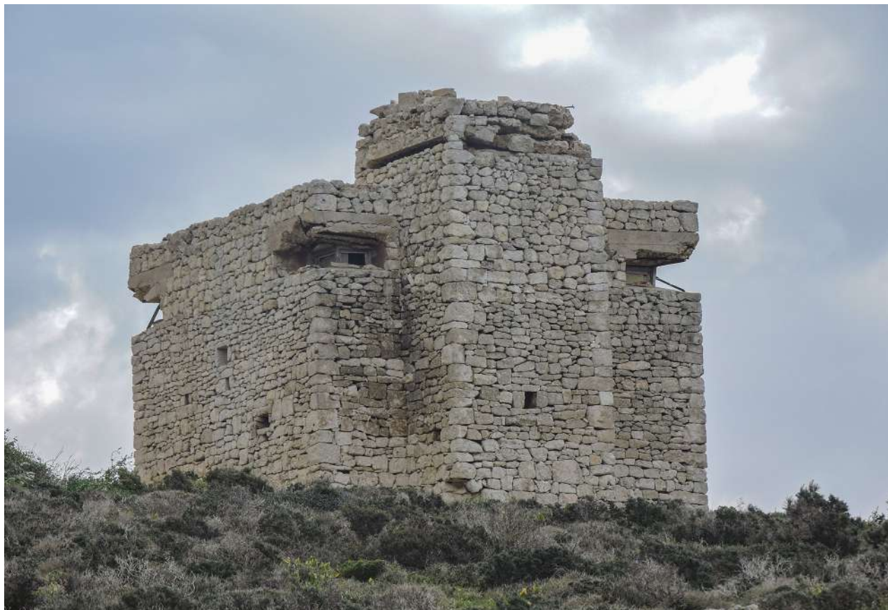
A squarish pillbox with a longish turret and four machine-gun portholes at Il-Qammieh.
